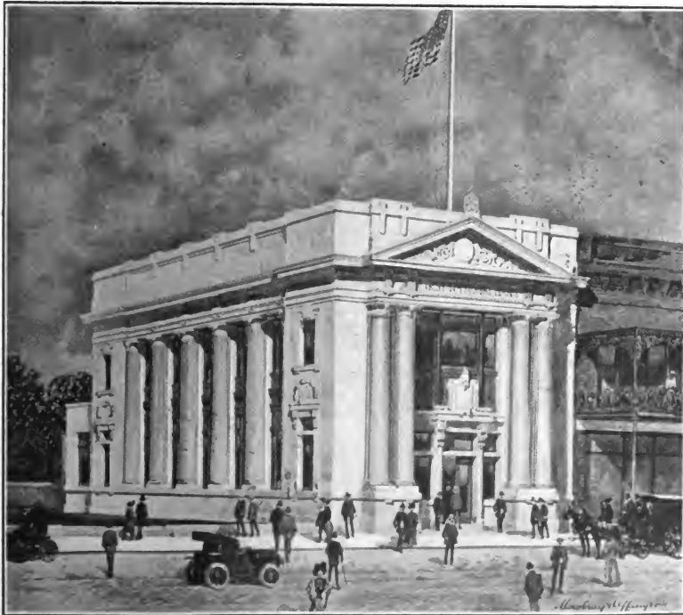
NEW BUILDING, FIRST NATIONAL BANK, PENSACOLA, FLA.
